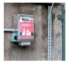
▶ 青洲英坭於廠房外指定吸煙區出入口設有語音自動播放裝置,提醒員工吸煙危害健康。 Infrared sensing audio reminder system was installed at the entrance of the designated smoking area to remind employees about smoking hazards.
